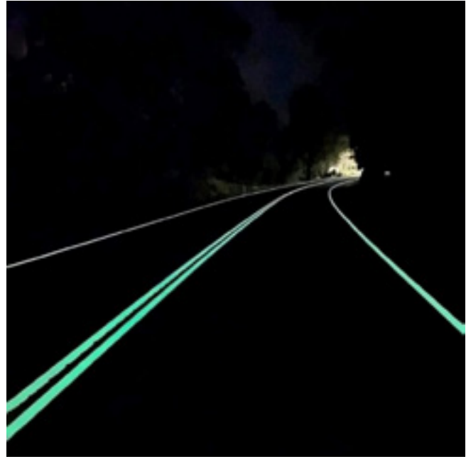
Figure 7. highlighting the effect of photoluminescent green glow paint, which glows in the dark for road and line marking. Source: author's contribution.
