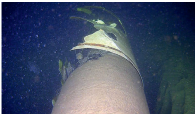
Fig. 3. The damaged offshore Balticconnector gas pipeline. Source: [8]
