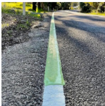
Figure 6. marking with green glow paint - photoluminescent/glow in the dark road & line marking. Source: author's contribution.
